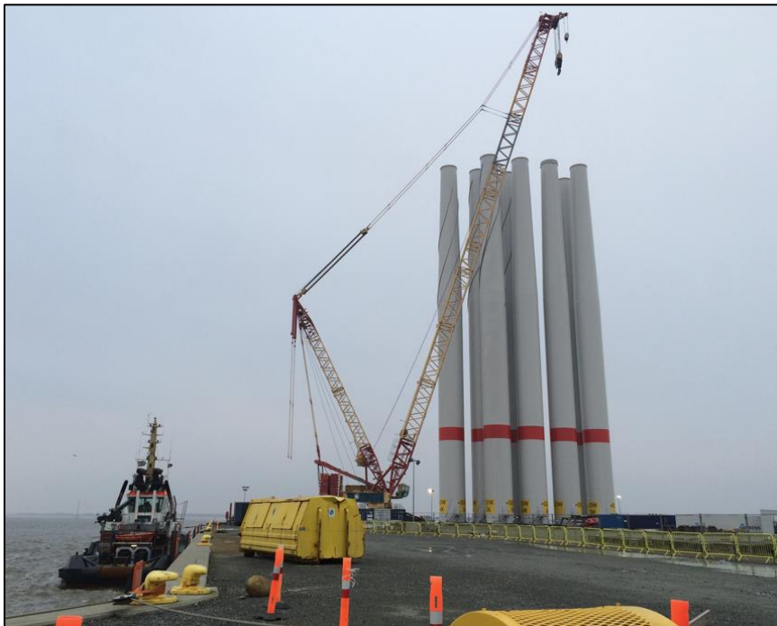
Figure 3.4-6. Typical lattice-boomed crawler crane
