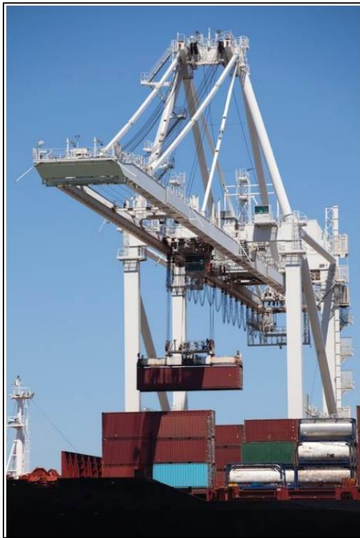
Figure 3.4-1. Container port crane
