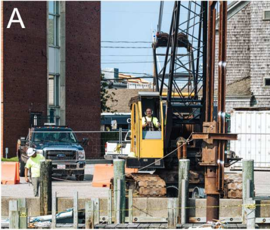
Figure 3. Picture of the impact (A) and vibratory (B) hammers used to drive the pile.
