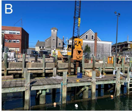
Figure 3. Picture of the impact (A) and vibratory (B) hammers used to drive the pile.
