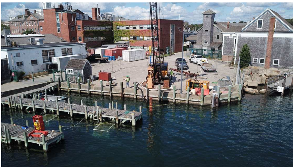
Figure 2. Aerial picture of the pile driving site off WHOI's dock showing the crane and cages at the near site.
