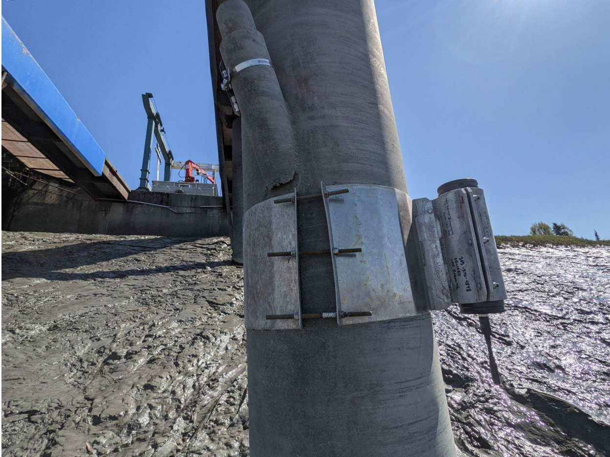
Figure 21: Kasilof ST500 dock piling welded bracket deployment, June 2021.
