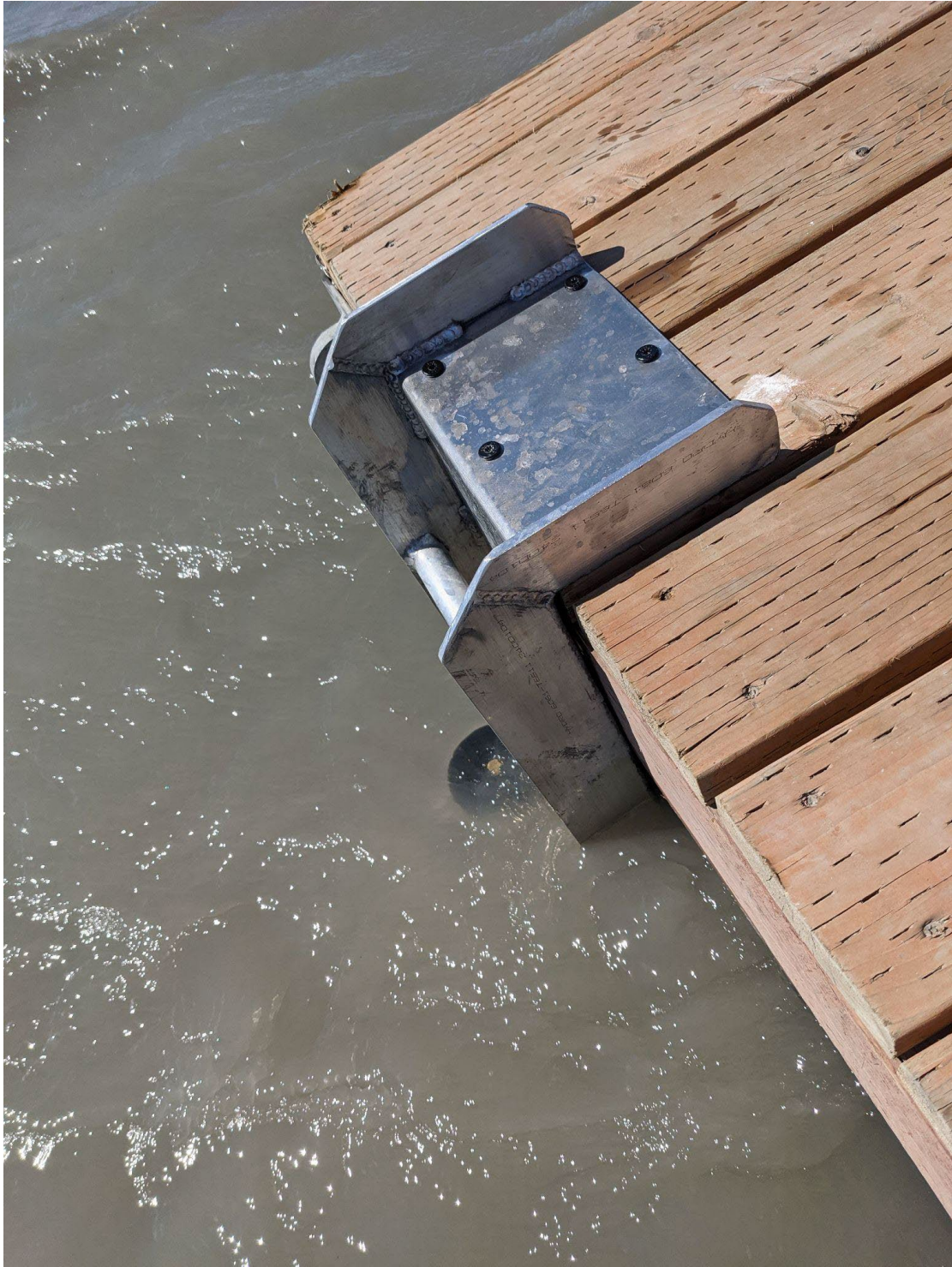
Figure 17: Kenai River ST500 floating dock deployment, June 2021.
