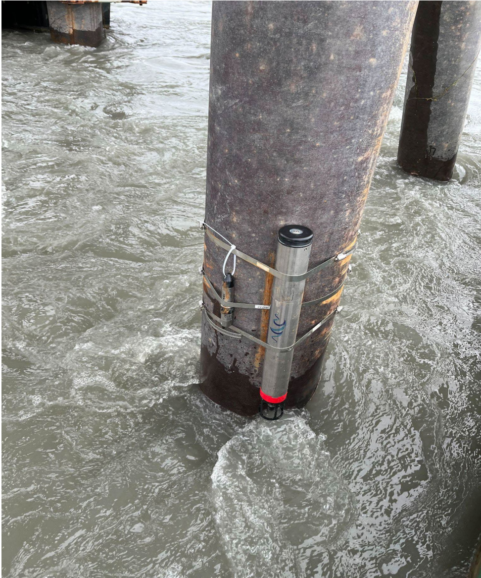
Figure 22: ST600 hoses clamped to a dock piling in the Kasilof River.
