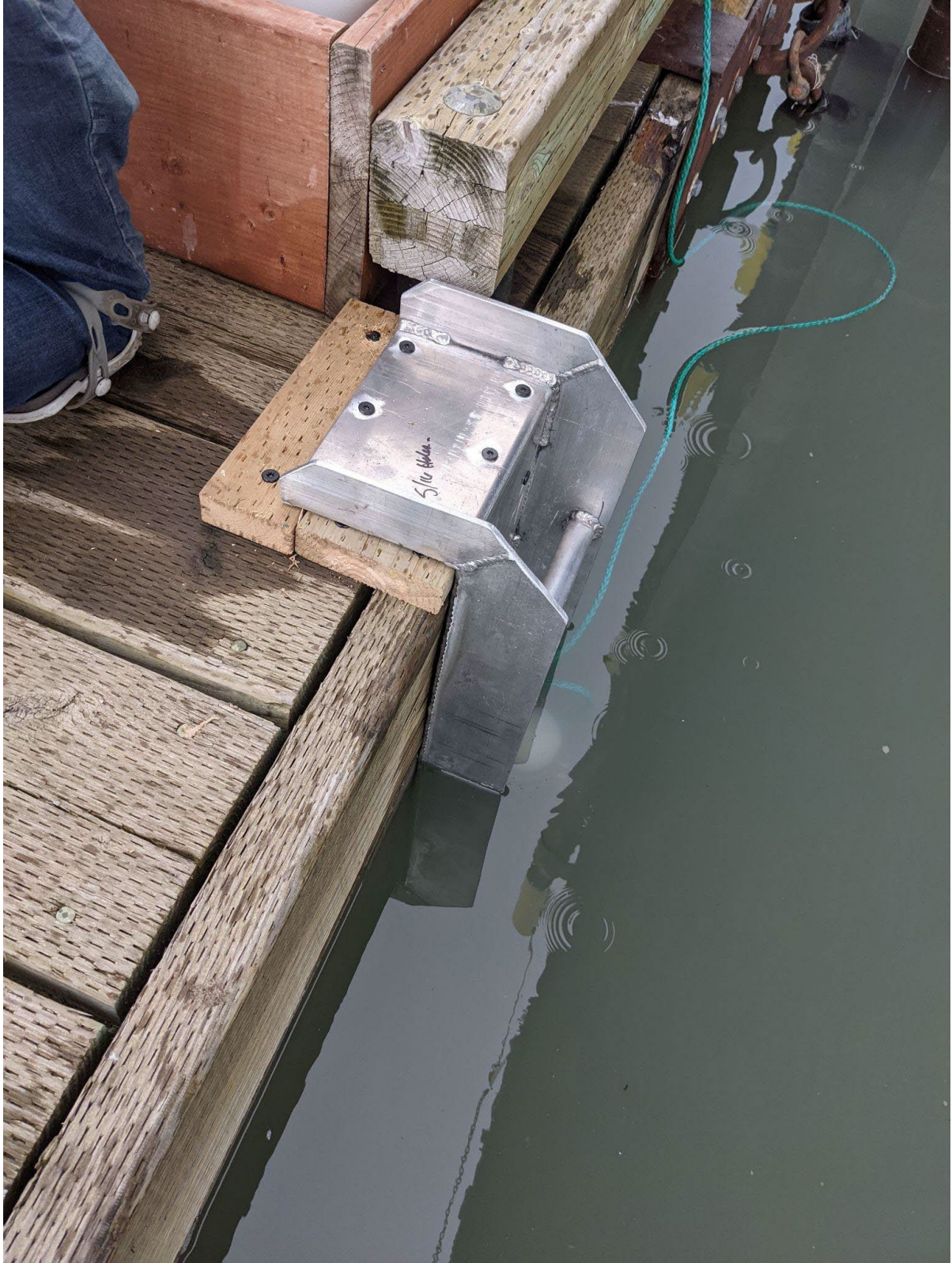
Figure 16: Cannery Lodge floating dock deployment, June 2021.
