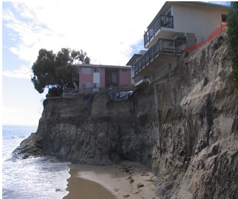
Figure A-1: Effects of shoreline erosion in Isla Vista, CA. Image source: U.S. Geological Survey
