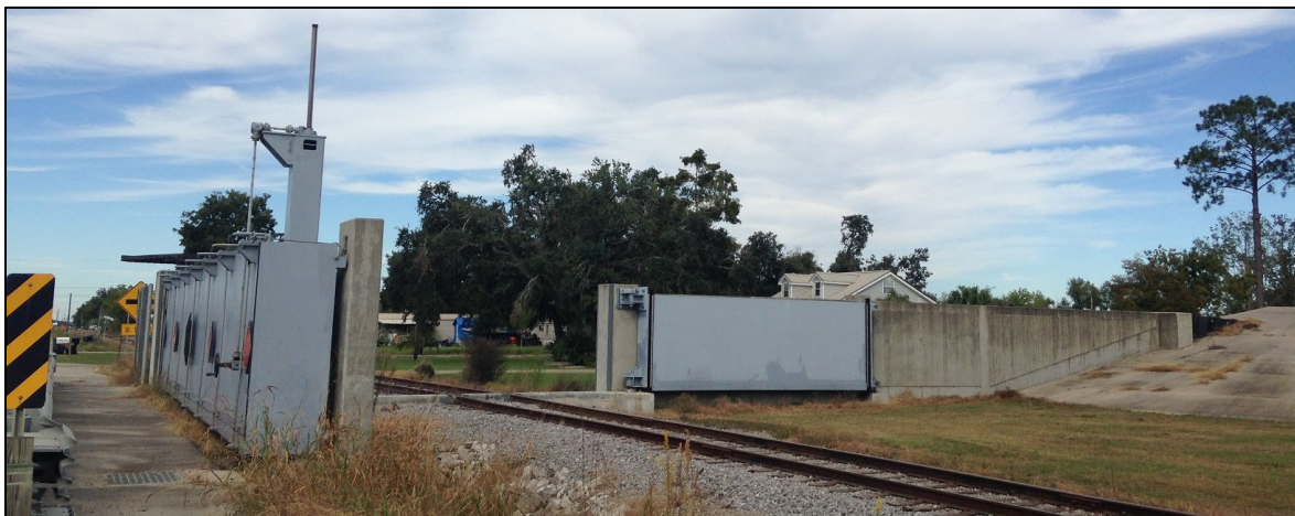
Figure 4.2. Floodwall in Plaquemines Parish
