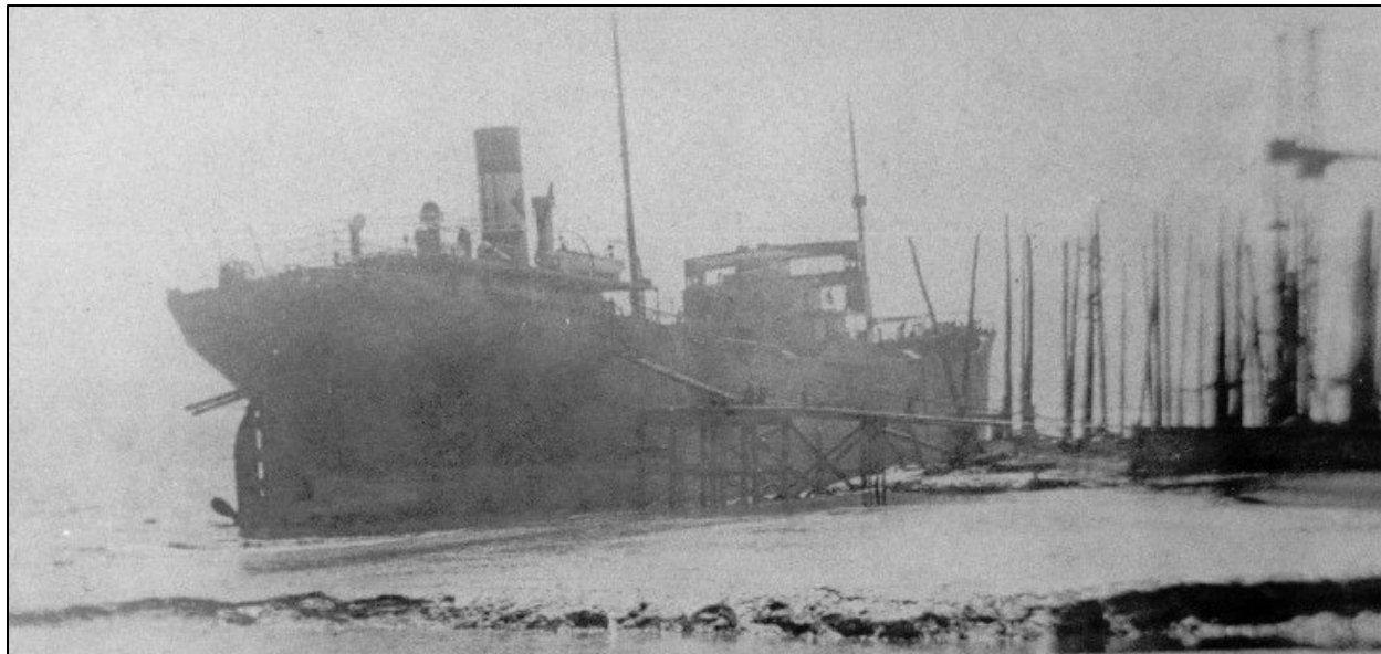
Figure 7-270 Stern view of Onokia in 1925 fitting out on the River Humber at Livingstone & Cooper Shipyard in Hessle, UK.
