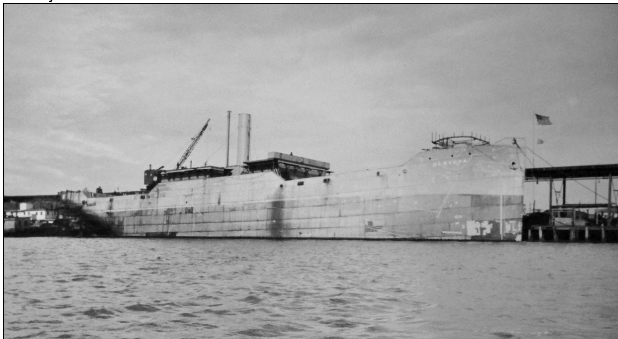
Figure 7-217 Chetopa still under construction at Newark Bay Shipyard on 27 September 1918.
