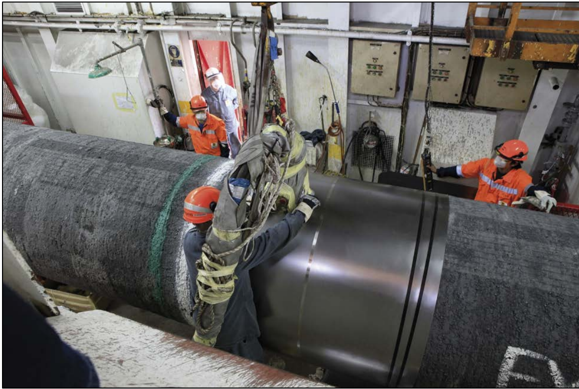
Figure E.4. Polyurethane foam being pumped into a joint mold.
