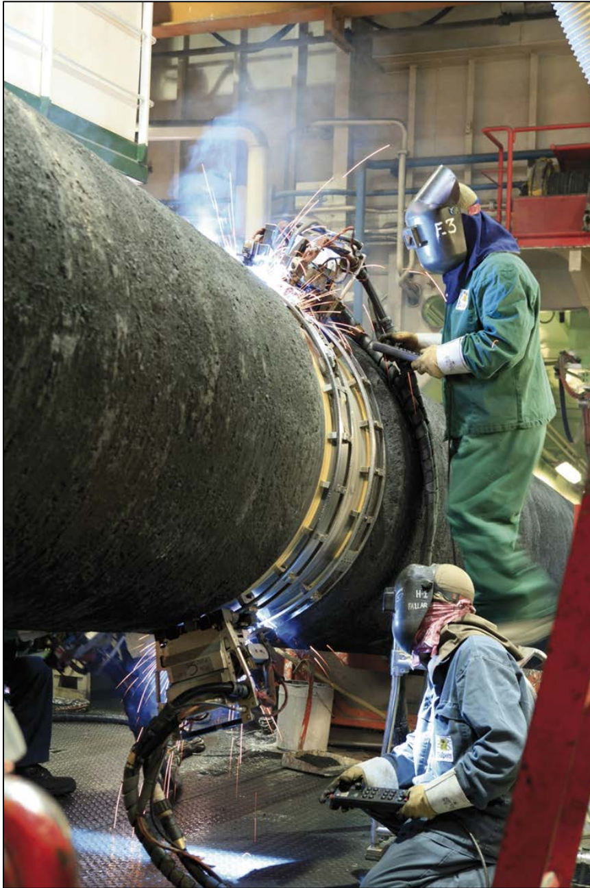
Figure E.3. Automatic welding of a pipeline.
