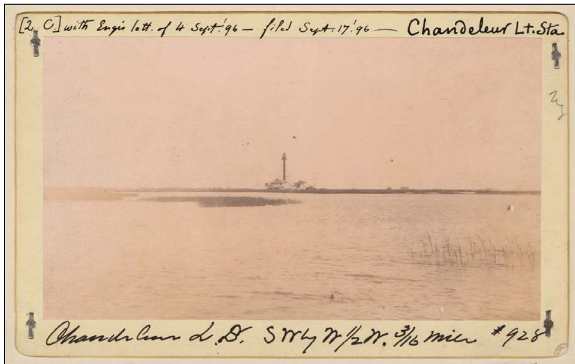
Figure 65. Chandeaur light station; image taken 4 September 1896.
