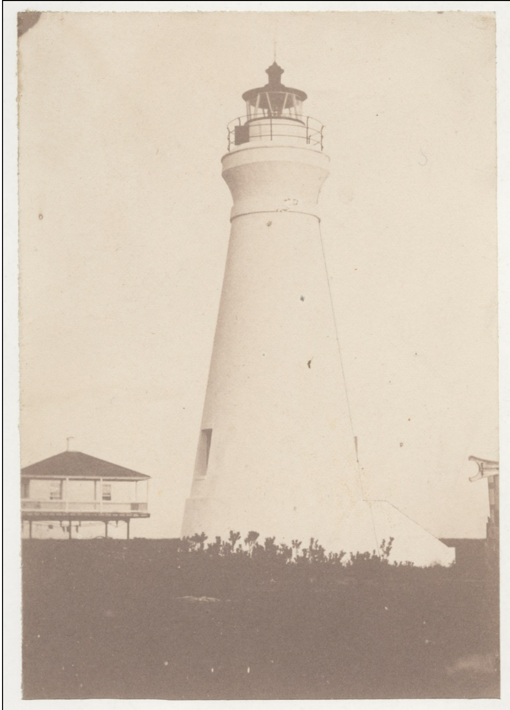
Figure 62. Photograph of 1856 Chandeleur light station taken before the October 1893 hurricane. (Courtesy of NARA.)
