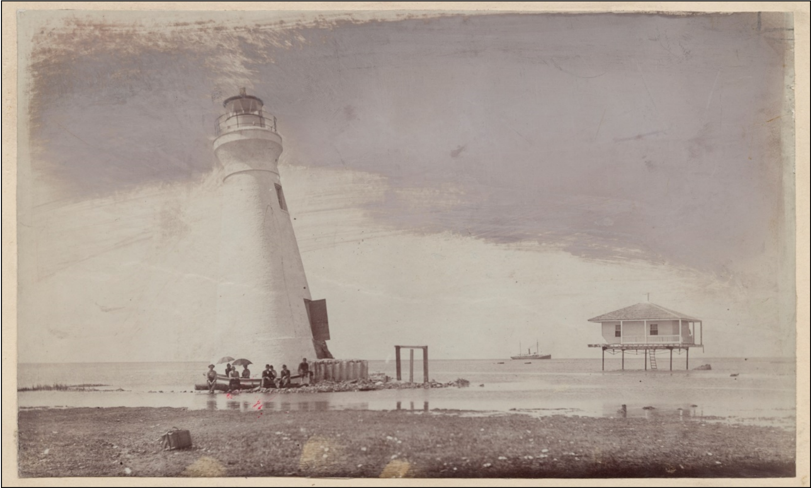
Figure 63. Photograph of Chandeleur lighthouse taken after the October 1893 hurricane. (Courtesy of NARA.)
