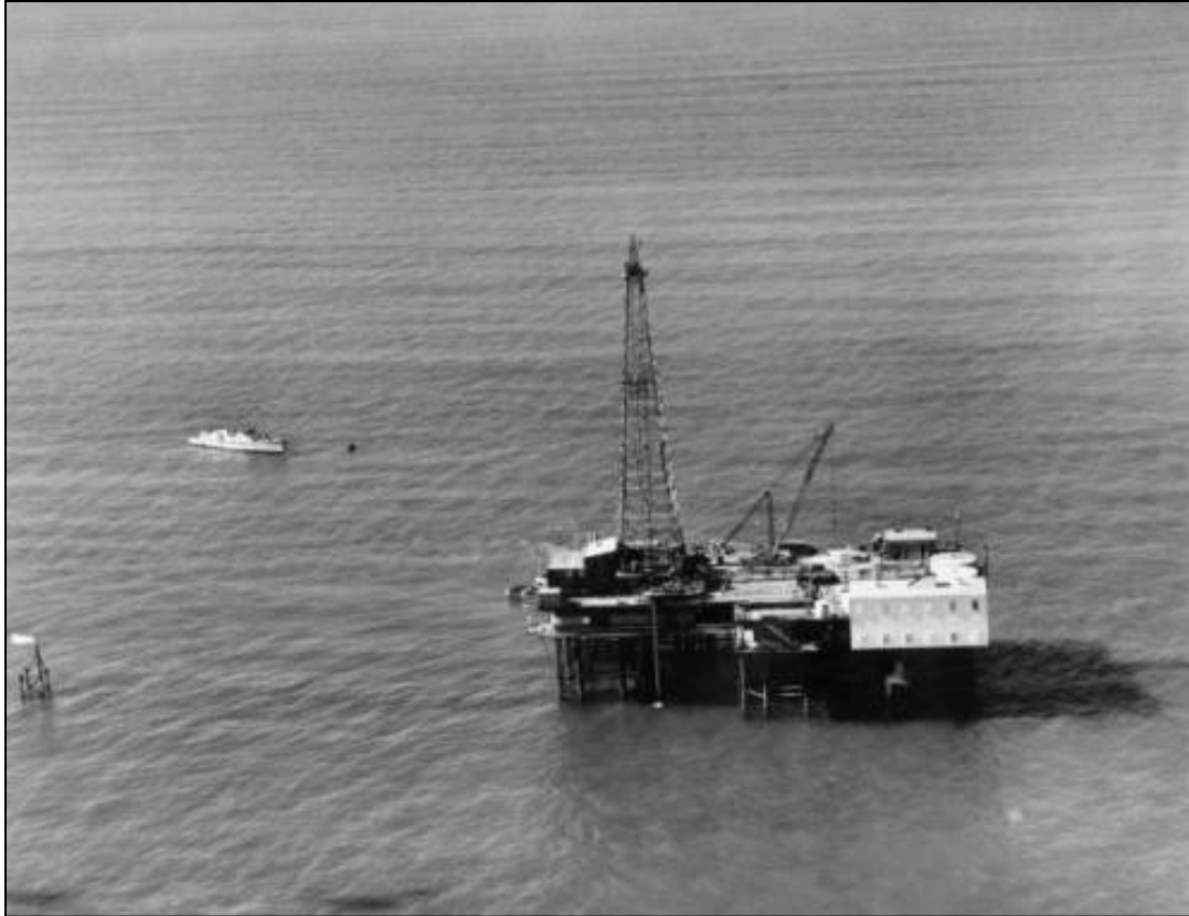
Figure 113. Humble #36 showing quarters, storerooms, storage tanks and support vessel, October 1948. (Courtesy of Standard Oil [New Jersey] Collection.)
