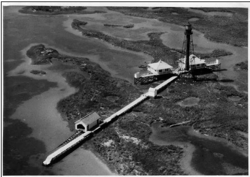
Figure 127. Aerial view of Chandeleur Lighthouse complex, date unknown. (Courtesy of USCG.)
