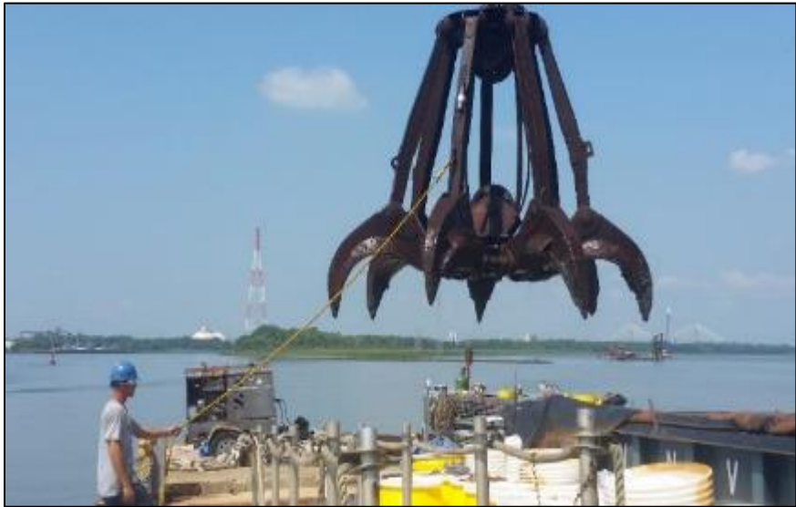
Figure 220: Mechanized recovery grapple with USBL transducer attached.
