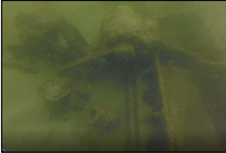
Figure 174. Engine bed with attached generators at HP S4B trawler site.
