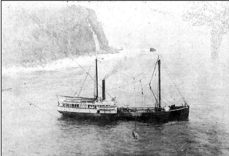
Figure 33: SS *Kaula* (RN375) moored and rigged to receive cargo from the overhead cable system, at Hakalau Landing on the Hāmākua coast, 1905. (Hawai'i State Archives)
