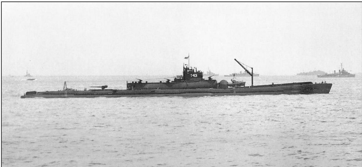
Figure 69: Image of Japanese submarine *I-401*, showing watertight aircraft hangar (forward door open), Seiran aircraft being recovered by retractable crane. (*I-400 Class Submarine* 2017)
