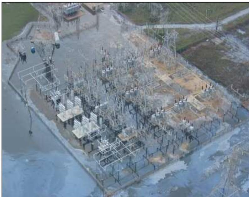
**Figure 137. Substation flooded by Hurricane Katrina.**
