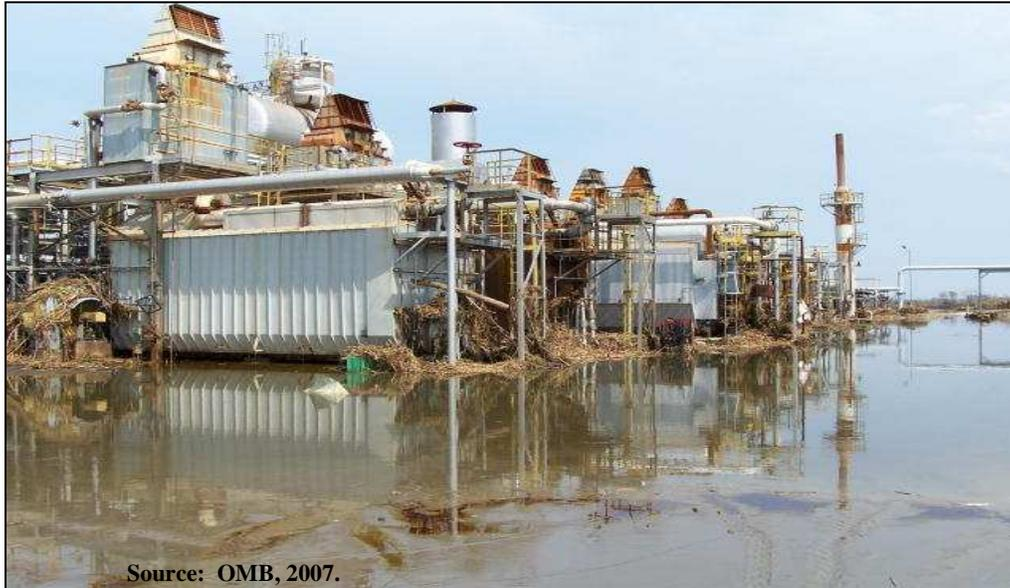
**Figure 89. Natural gas processing plant flooded by Hurricane Katrina.**
