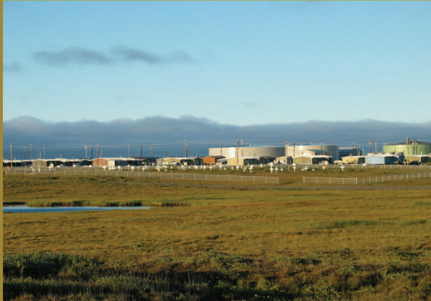
Government infrastructure and service-related employment is significant
