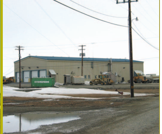
Public works building
