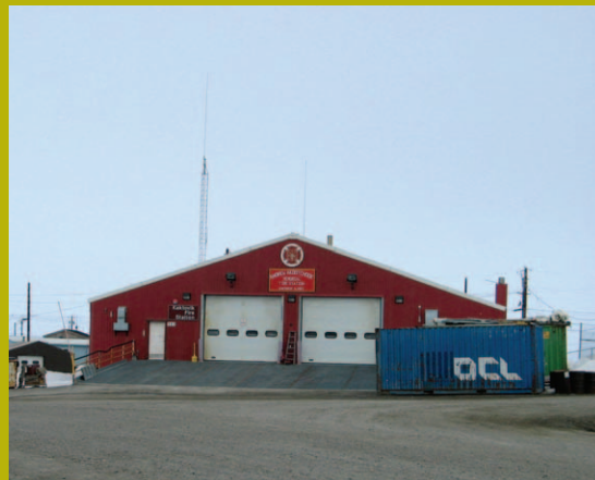
Kaktovik Fire Station
