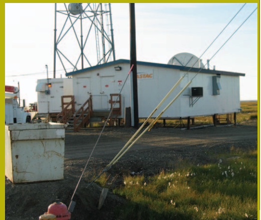
Arctic Slope Telephone Association Cooperative
