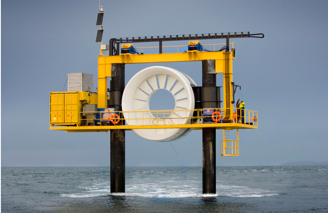
Figure 3-11: Installation of an open center current/tidal turbine.
