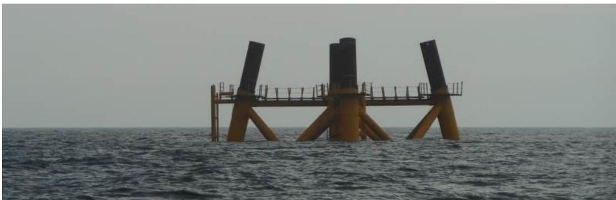
*Figure 1-4 Jacket with four driven piles*
