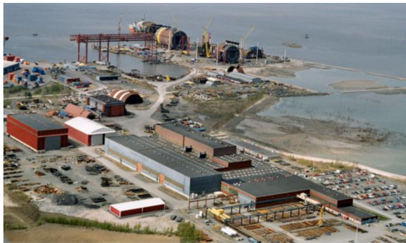
Figure 4-3. Hywind construction location in Pori, Finland (Technip 2013)
