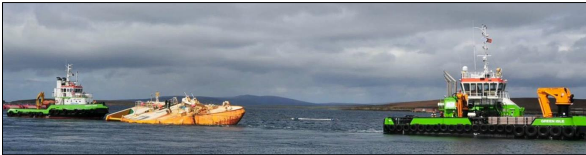
Figure 3-7. Wello Penguin Installation at EMEC by two multicat tugs (CEFOW 2015)
