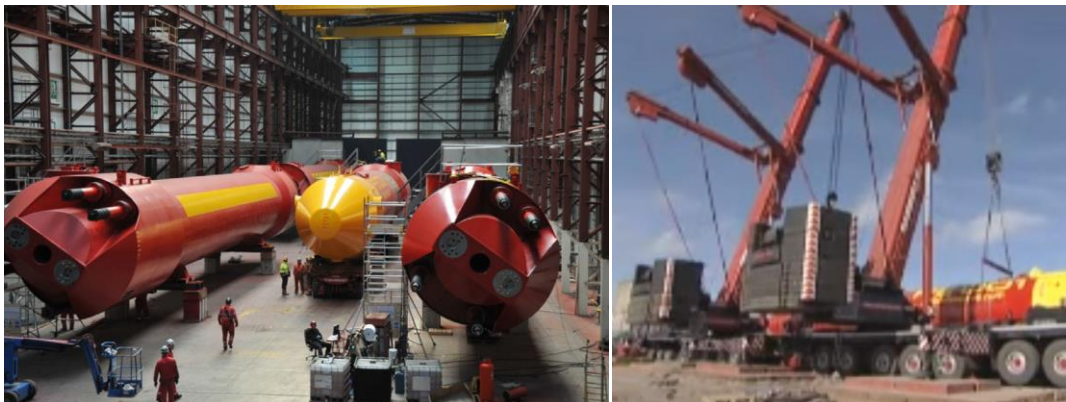
Figure 4-5. Pelamis device installation (Yemm et al. 2011)
