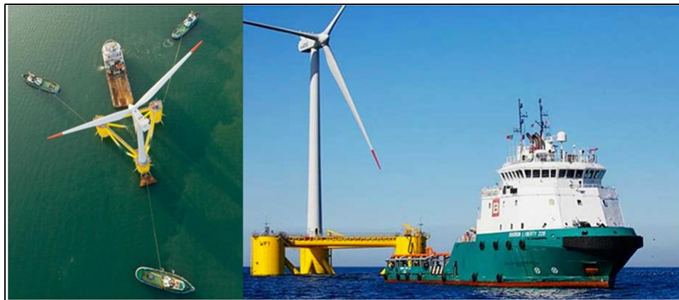
Figure 3-3. Semi-Sub demonstration project installation (WindFloat, 2014)
