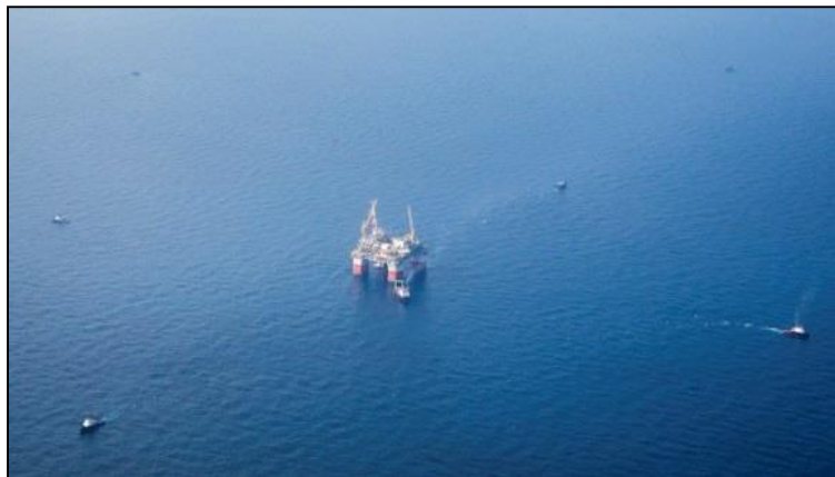
Figure 3-9. Installation of Semi-Sub FPU utilizing tugs in star formation (Crowley 2014)
