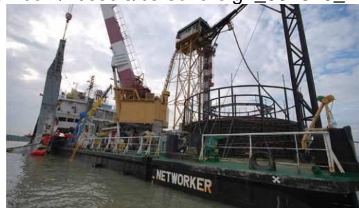
Cable Laying Barge 4 - CB Networker [ http://www.cablesm.fr/CB%20Networker.pdf ]
