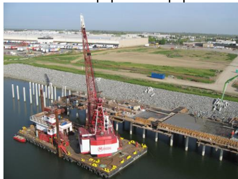
Crane Barge (700-1000 ton) 16 Manson Crane
