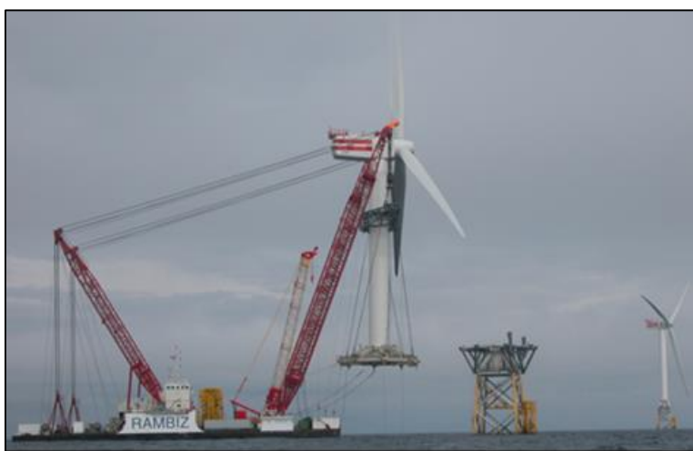
Figure 3-2. Floating Crane Barge Rambiz 3000 installing a wind turbine (Wind Energy The Facts, 2016).
