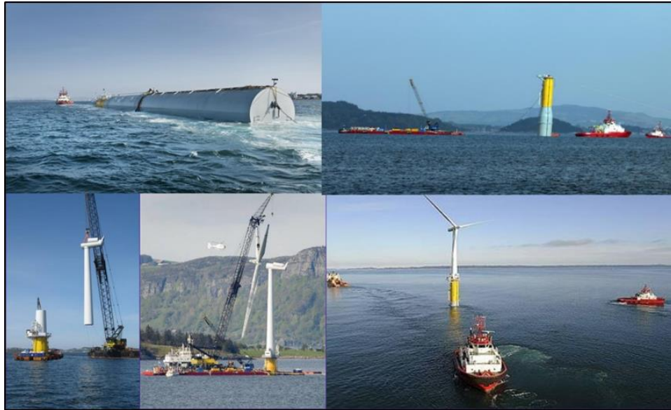
Figure 3-4. Spar demonstration project installation example (Hywind 2015)
