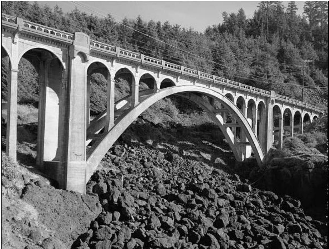
Figure 65. Rocky Creek Bridge, 1927, Depoe Bay vicinity, Lincoln County, Oregon. This is one of multiple coastal bridges designed by noted Oregon State Highway engineer Conde McCullough during the 1920s and 1930s. Photograph taken since 1968, exact year unknown (From Library of Congress 2013e).
