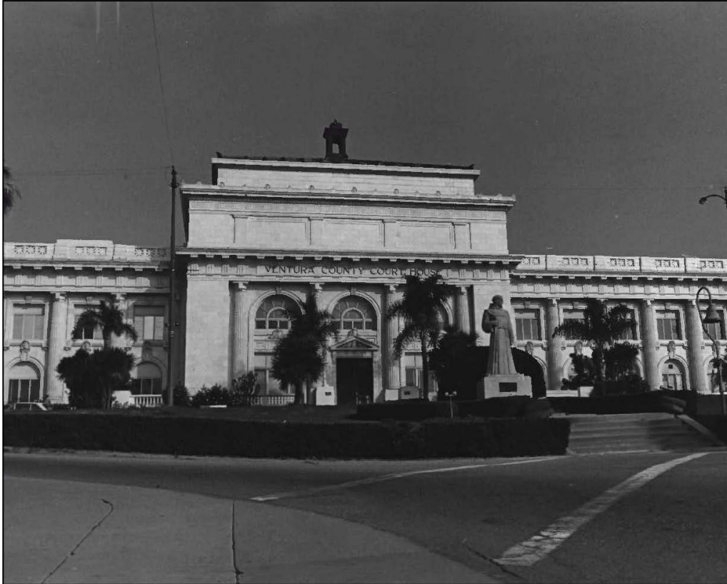
Figure 46. Ventura County Courthouse, 1912, Ventura, California (National Register # 71000211). Classical Revival-style courthouse built for Ventura County. Photographed in 1971 (From National Park Service 1971a)
