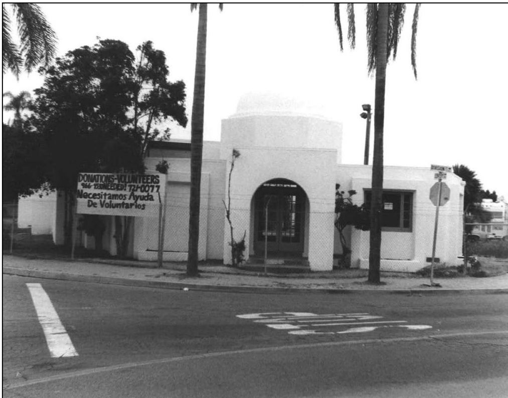
Figure 42. Americanization School, 1931, Oceanside, California (National Register # 94000311). A Moderne-style building with Islamic influences designed by master architect Irving Gill. Photographed in 1993 (From National Park Service 1994).
