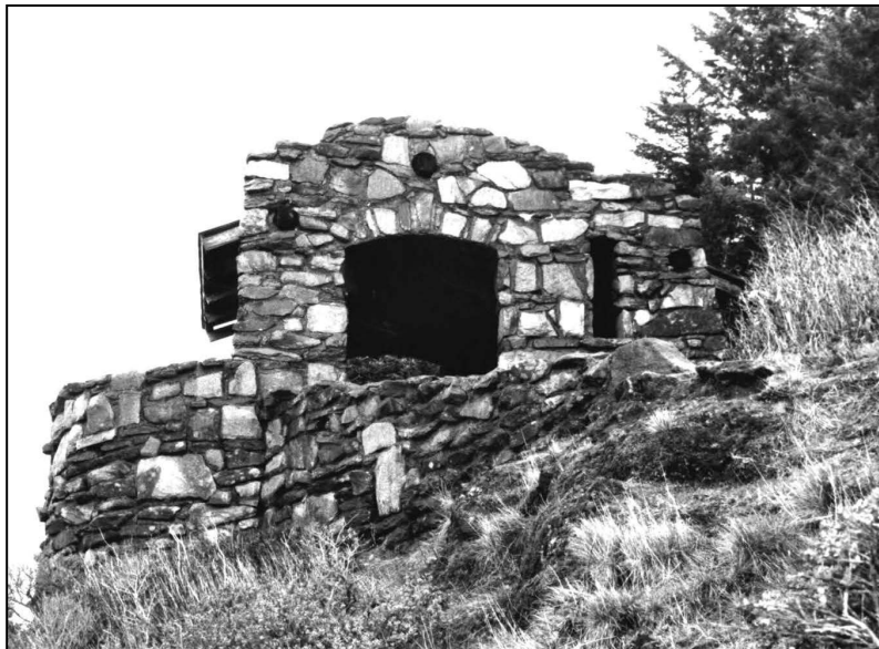
Figure 63. Cape Perpetua Shelter and Parapet, 1933, Siuslaw National Forest, south of Yachats in Lincoln County, Oregon (National Register # 88002016). Created by the Civilian Conservation Corps (CCC), the shelter and parapet are the only stone structures built atop Cape Perpetua. They are also the only remaining recreation sites developed by the CCC at the Cape. Photographed in 1988 (From National Park Service 1989).
