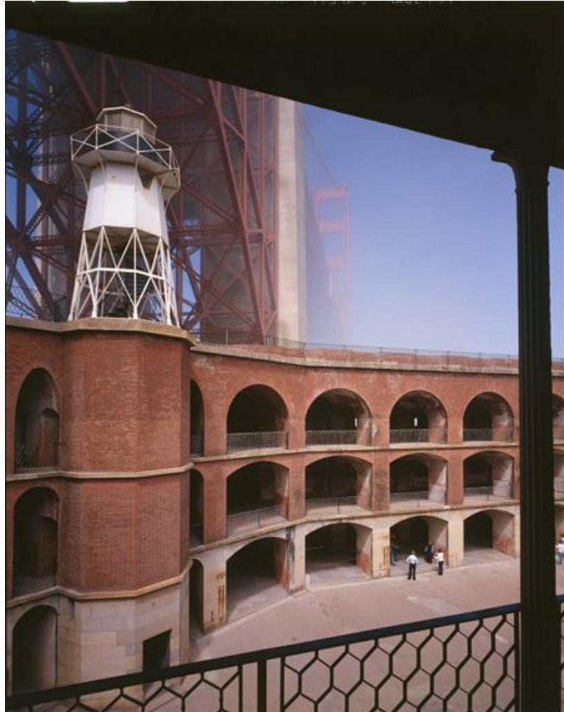
Figure 52. Fort Point 1861, San Francisco, California (National Register # 70000146). A masonry fortress, this National Historic Site features a courtyard surrounded by three stories of tiered brick arches and an octagonal metal lighthouse capping the northwest tower (From Library of Congress 2013c).
