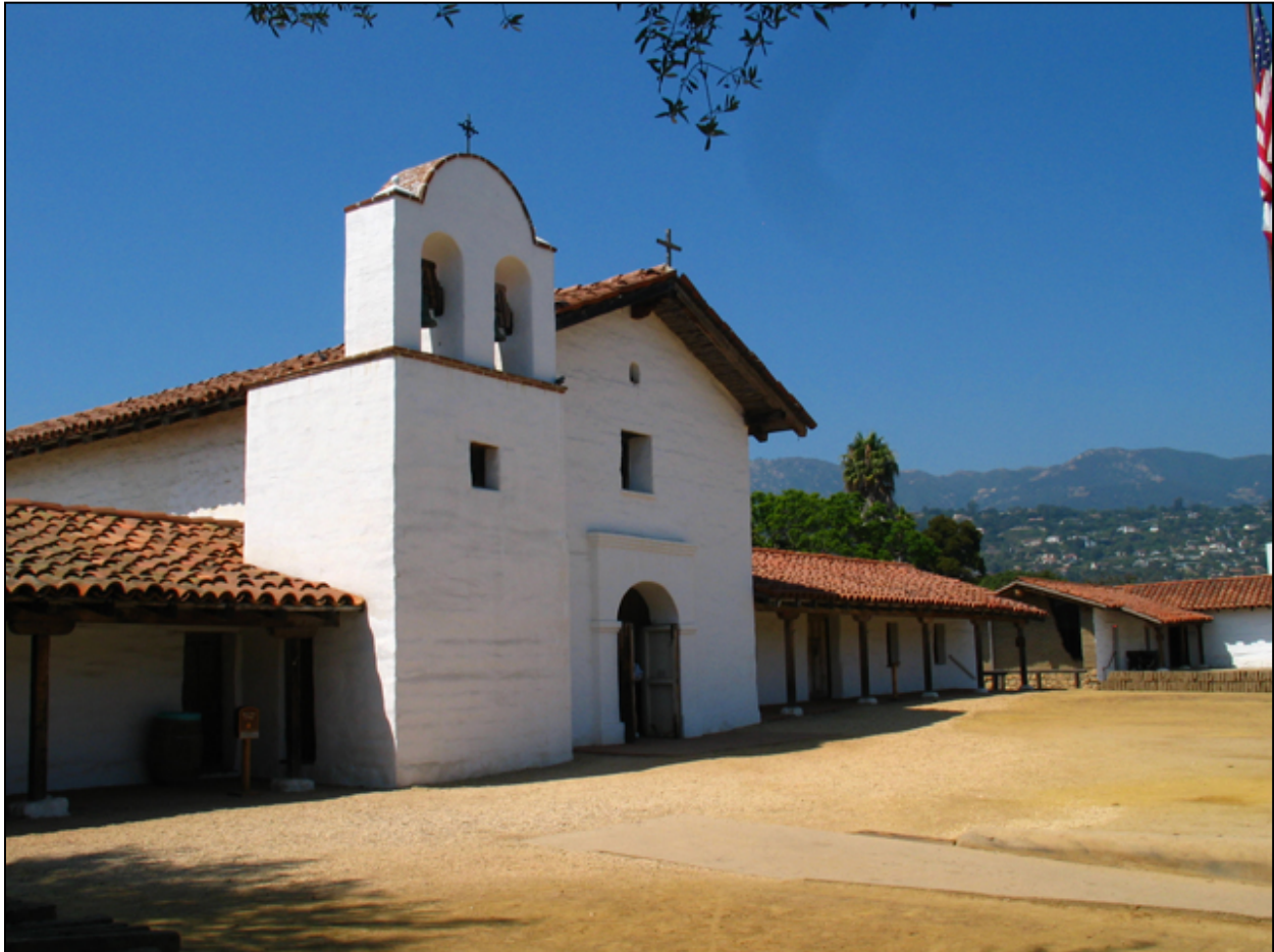
Figure 51. El Presidio de Santa Barbara, 1788–1797, Santa Barbara, California (National Register # 73000455). This Mission-style fortress, now a California State Park, includes multiple extant Spanish adobe structures (From California Department of Parks and Recreation 2013b).
