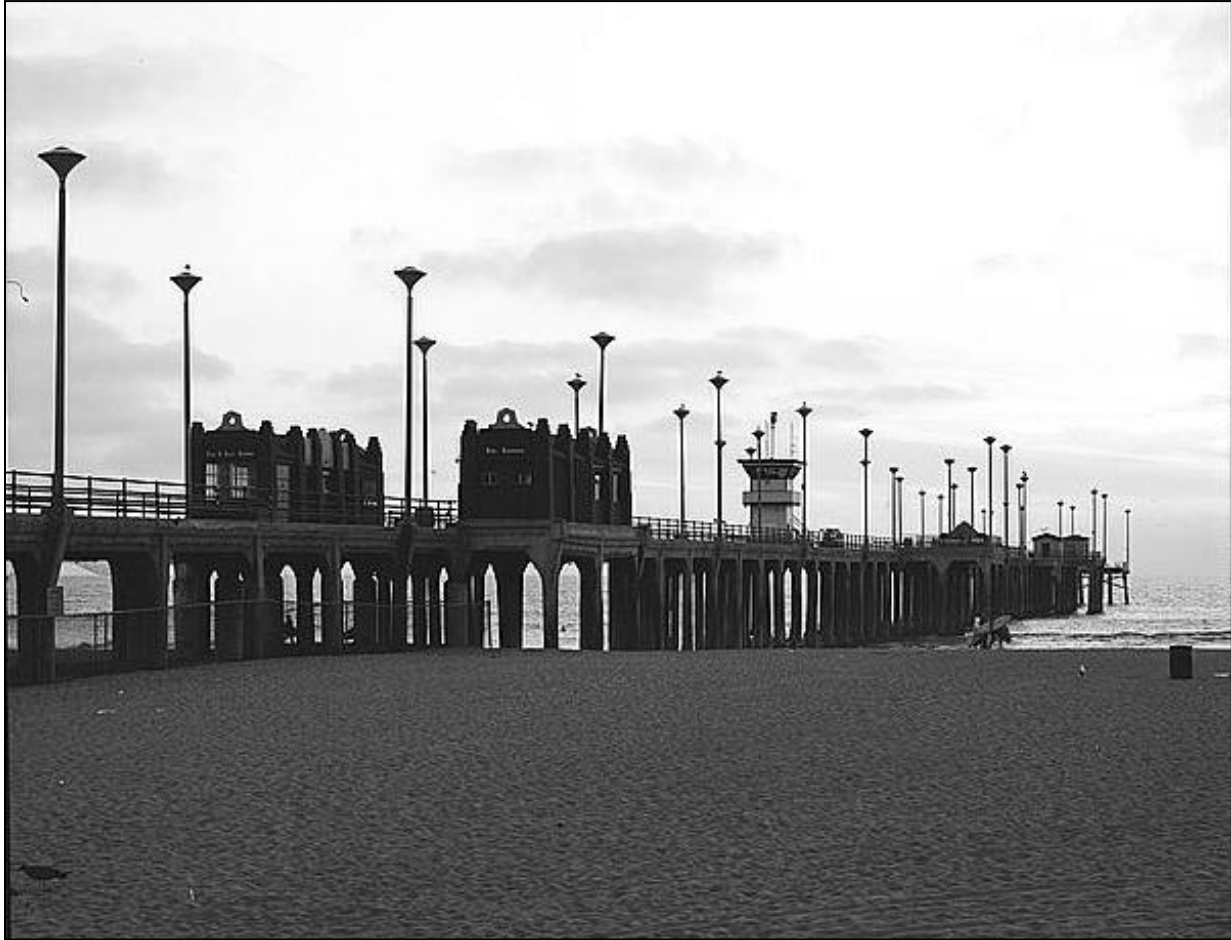
Figure 59. Huntington Beach Municipal Pier, 1930, Huntington Beach, California (National Register # 89001203). A historic district with Art Deco-style pier buildings. Photographed in 1989 (From Library of Congress 2013d).
