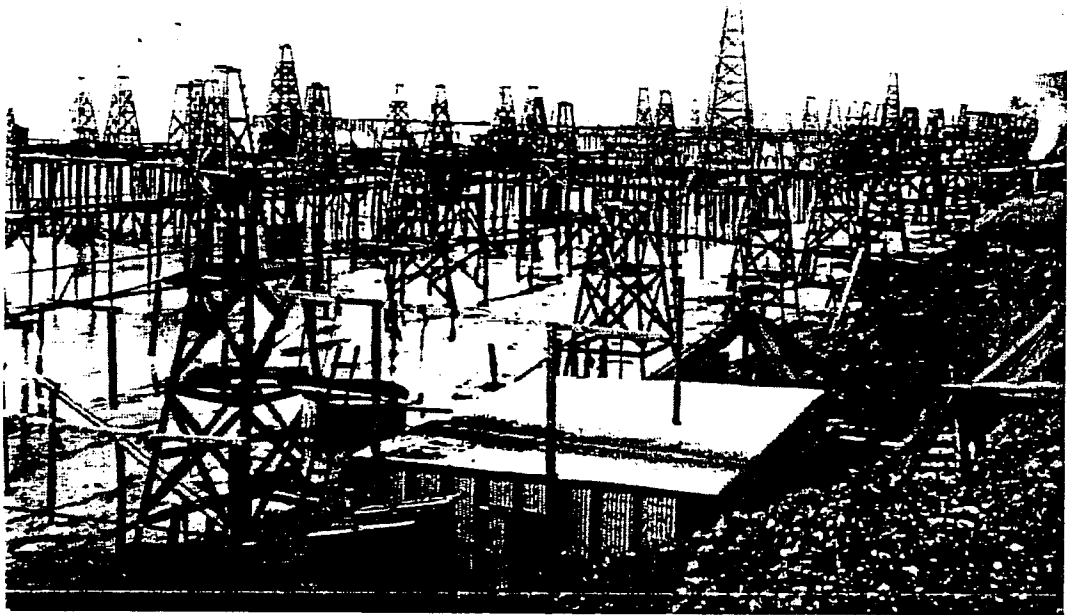
Photo 1: Summerland oil derricks (1930). Reprinted from Franks and Lambert (1985).
